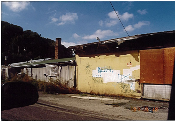
The Noji Gardens site before...
